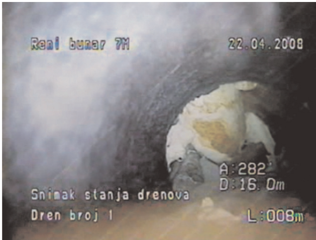
Fig. 5. Lateral filled with aquifer material.
